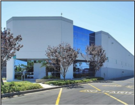
Prologis Targeted US Logistics Fund South Bay Distribution Center Rancho Dominguez, CA
